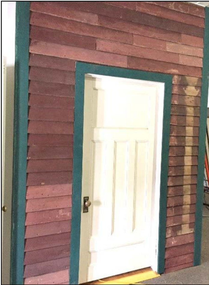
Original siding and constructed trim surrounding a 5-panel door
