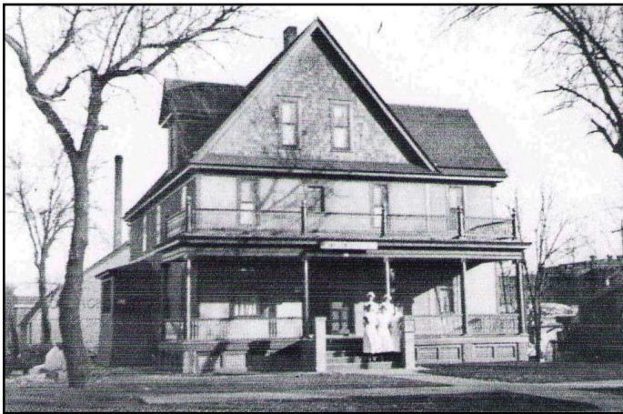
A photograph of the Vermillion Hospital in the 1920's and a Sanborn fire map of its footprint.
