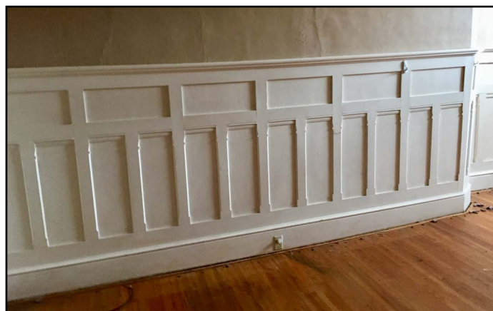
View of the white painted wainscoting
